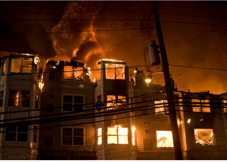
AVALON AT EDGEWATER APARTMENT COMPLEX EDGEWATER, NEW JERSEY
